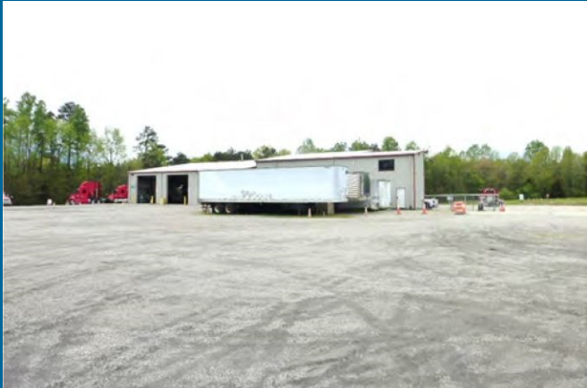
VIEW OF THE REAR ELEVATION OF THE SUBJECT PROPERTY
