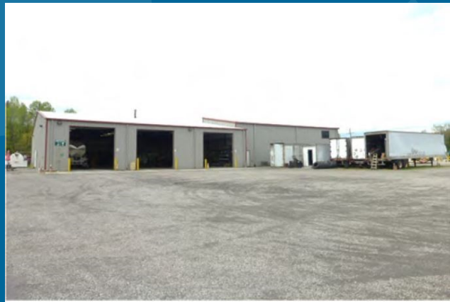
ANOTHER VIEW OF THE REAR OF THE SUBJECT PROPERTY
