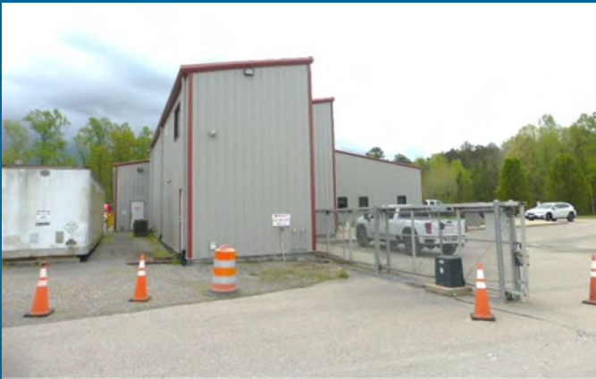
VIEW OF THE SIDE ELEVATION OF THE SUBJECT PROPERTY
